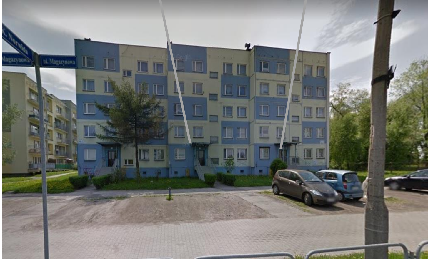
Fig. 3. Residential building in Ruda Śląska, Magazynowa Street
